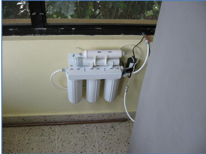
Figure B-1: Filter for Ice Machine
