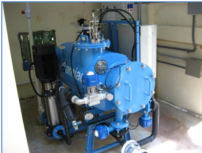
Figure A-8: Filter for Water after Concrete Tank
