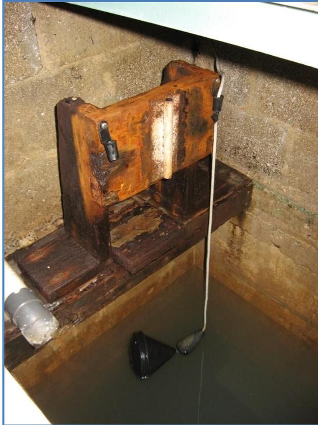
Figure A-7: Buoy Water-level Sensor in Concrete Tank
