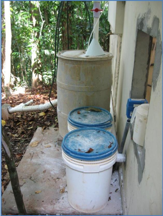
Figure A-10: Chlorine Powder (blue lid) and Chlorine Mixing Barrel (grey)
