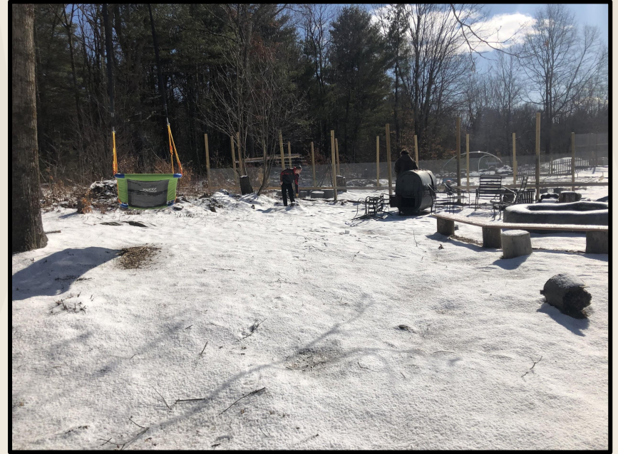
Kitchen Build Area
