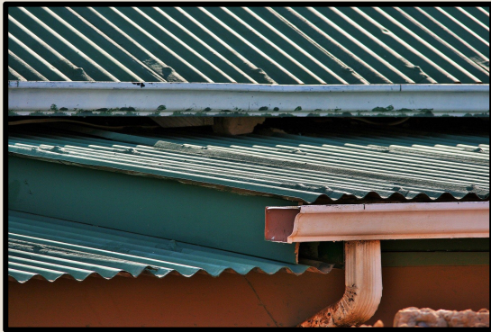
Corrugated Roofing Panels with Gutter
