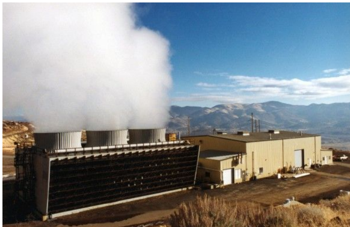
[109] Image Courtesy of the University of Michigan: Image of a geothermal power plant in Nevada,
