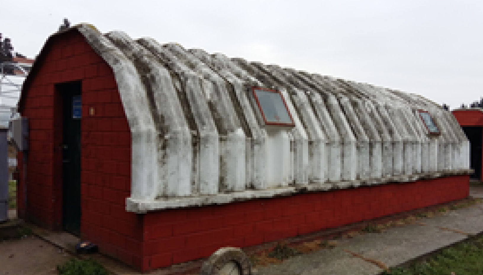
Figure 12: Building to be constructed into snail farm at AFS
