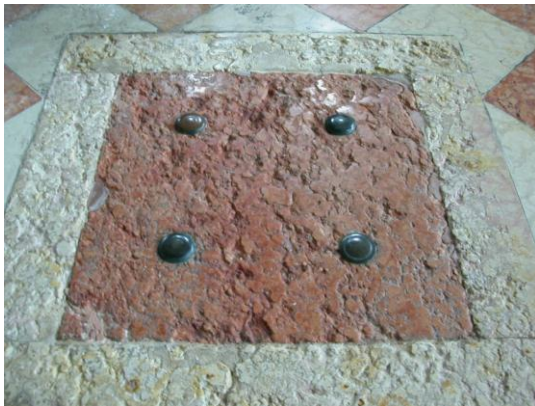
Figure 14: Examples of Holes & Joint Gaps
