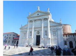
The façade of the church.
