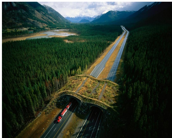
Figure 9: Wildlife Overpass in Banff National Park (Alberta, Canada) [37].
