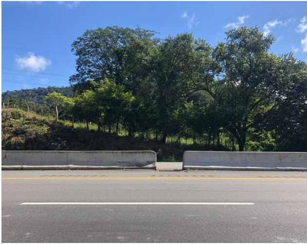
Figure 20: Current Accessibility to Crossing Animals through Jersey Barriers.
