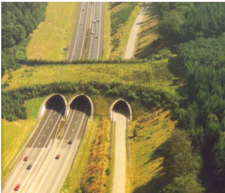
Figure 11: Aerial Image of the Ecoduct de Woeste Hoeve (The Netherlands) [41].
