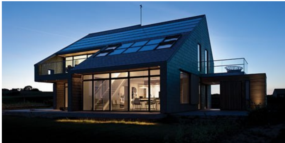
Figure 2: Net-Zero Energy Home in Aarhus, Denmark (Hansen, Ellen 2010).
