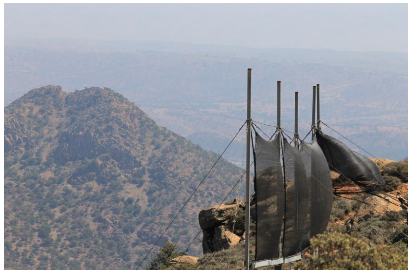
Figure 15: Detached fog nets from frames due to high winds
