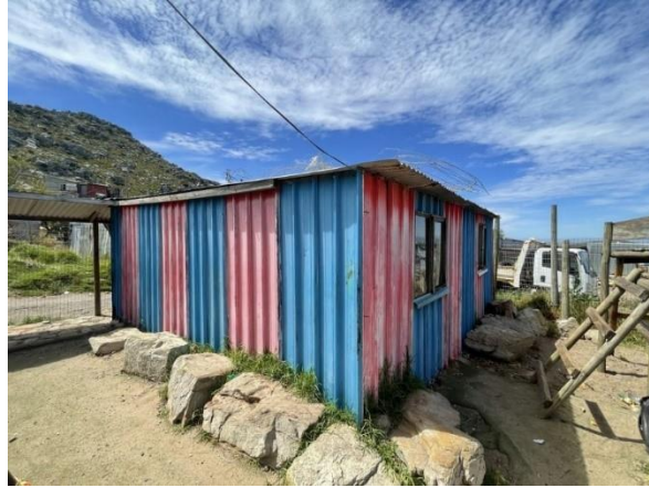
Figure 3: The outside of a building in a Red Hill ECD center
