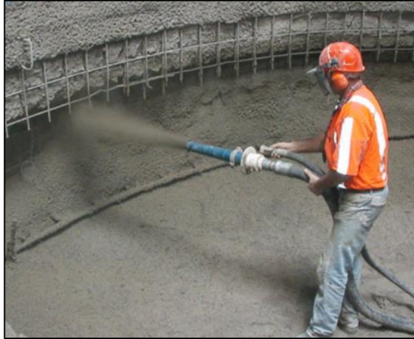
Figure 12: Sprayed Concrete (New Austrian tunneling method (natm) (n.d.)).
