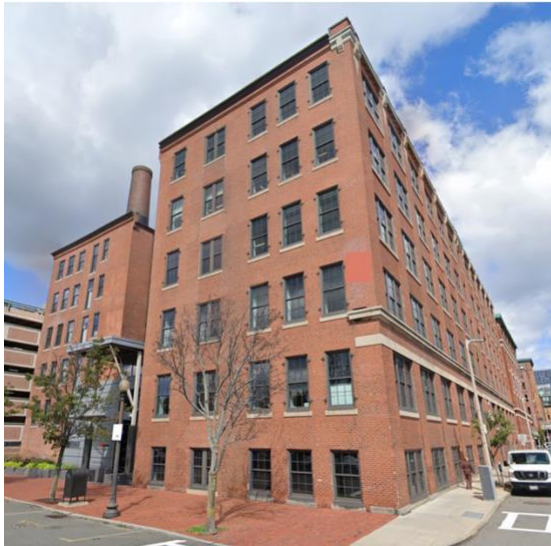
Figure 4.1: Exterior of the Case Study Building
