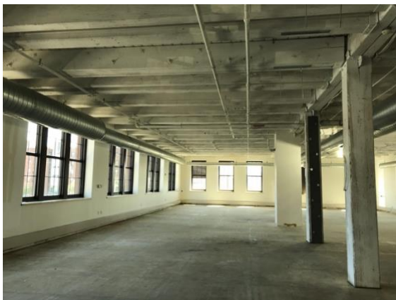
Figure 4.2: Interior of the Case Study Building
